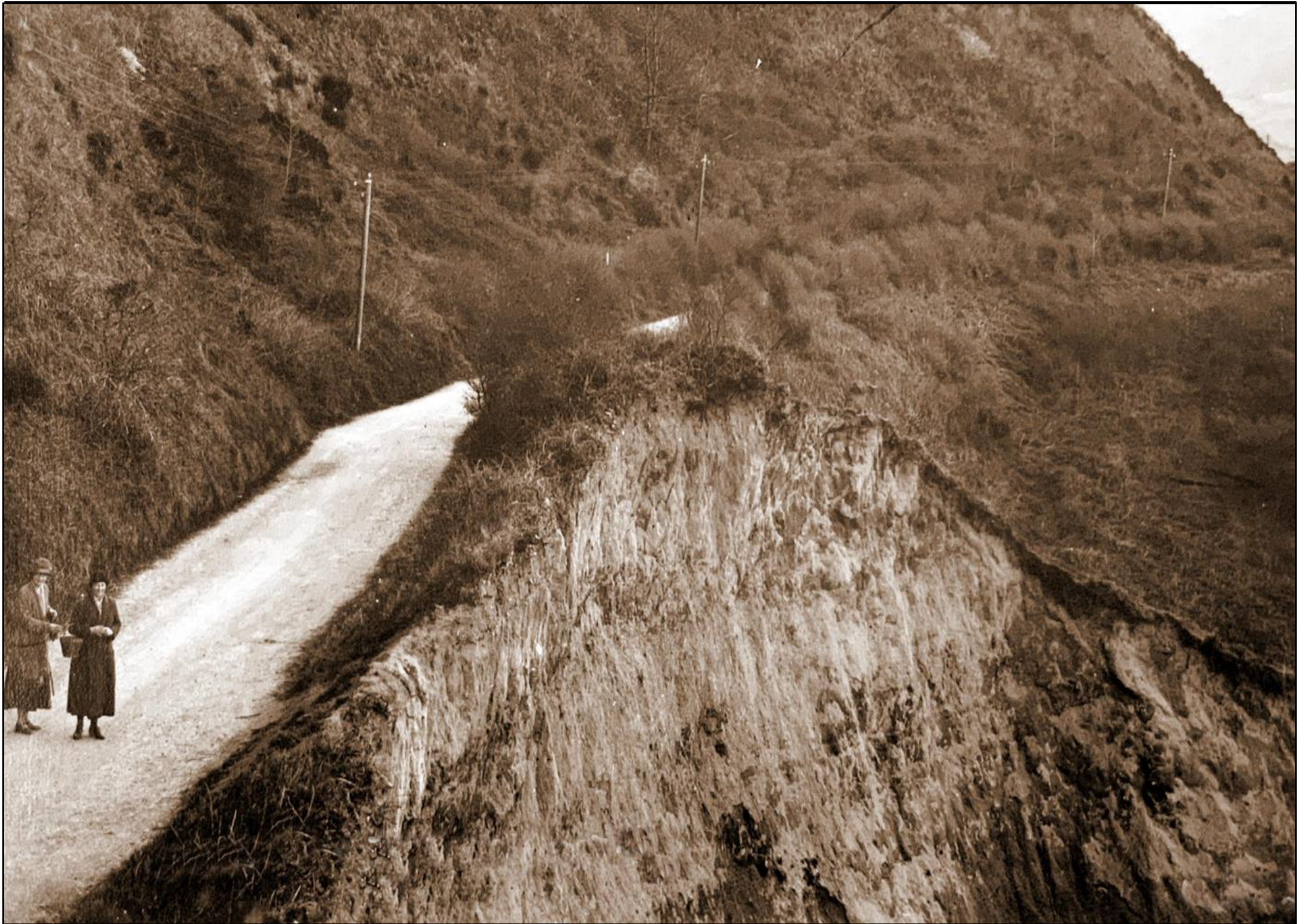
In May 1924 as a result of torrential rain the road linking Charmouth with Lyme Regis sank considerably as seen in this photograph.
